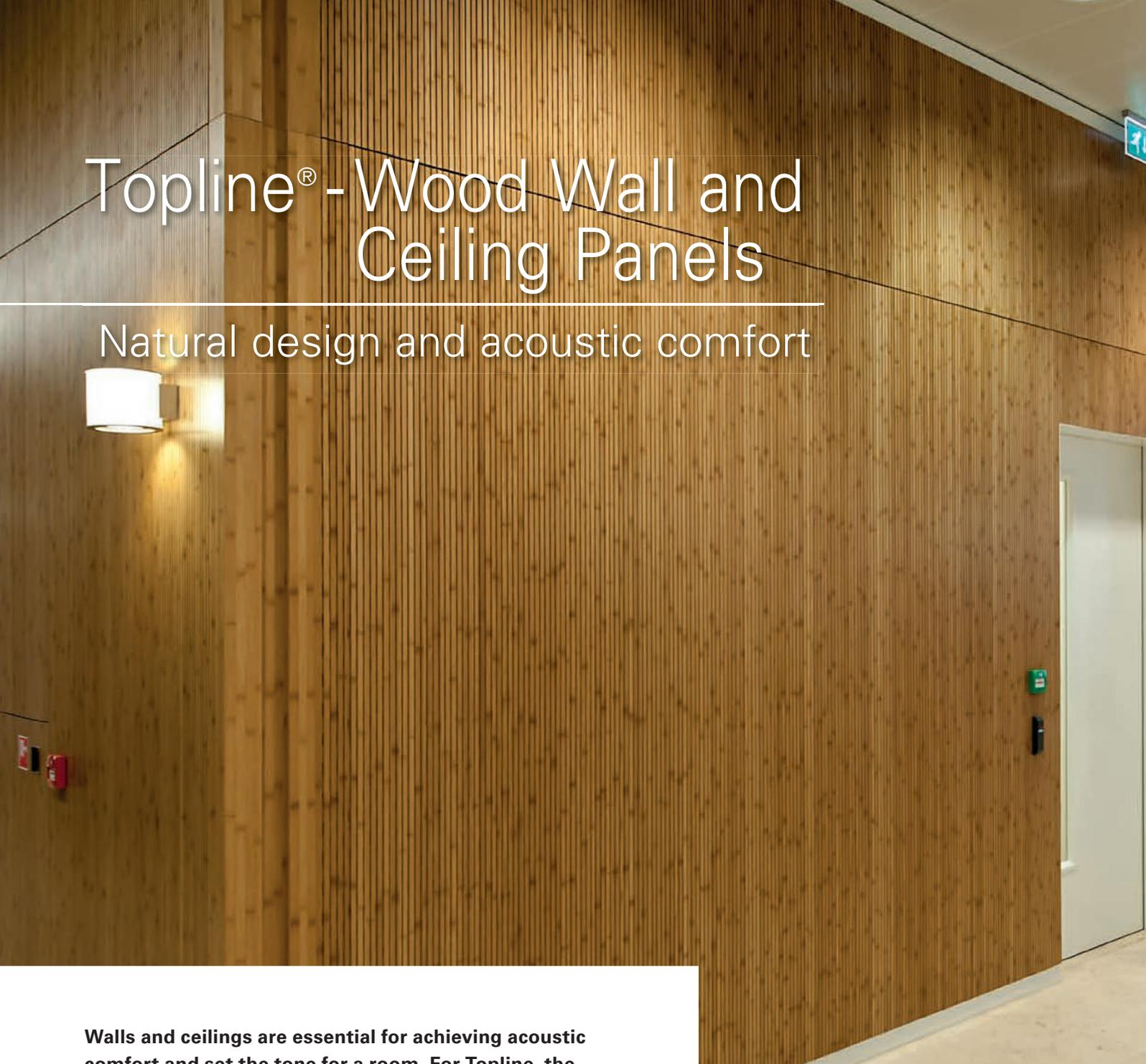
**Walls and ceilings are essential for achieving acoustic comfort and set the tone for a room. For Topline, the combination of sound reflection, sound diffusion and sound absorption can be fully coordinated with the requirements of the room in question. The visible side shows symmetrical grooves, while the other has a perforation design that enables sound energy to pass through.**
